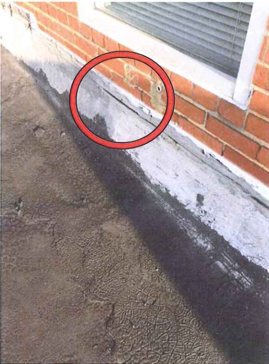
Elizabeth Hager Center: Typical Flashing Damage (cracked, broken, open)
