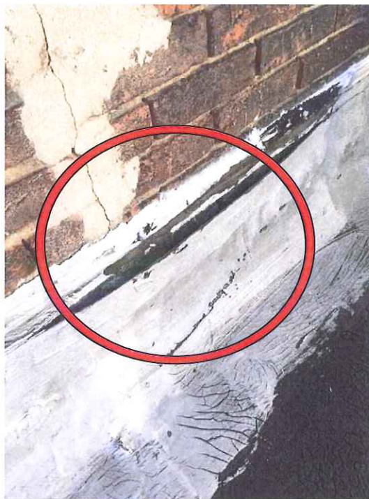
Elizabeth Hager Center: Typical Flashing Damage (cracked, broken, open)
