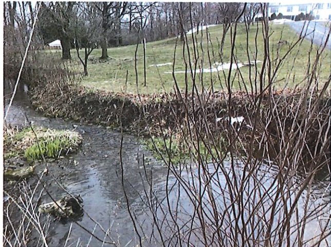
Photo 1. Existing conditions show a minimal vegetative buffer that consists of shallow rooting vegetation allowing for erosion.
