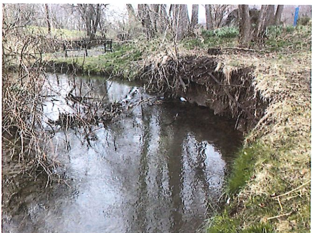
Photo 2. Existing conditions consist of an incised channel that is actively eroding and encroaching on nearby infrastructure.
