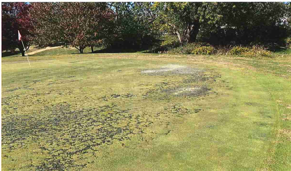
Hole No. 5 current condition.
