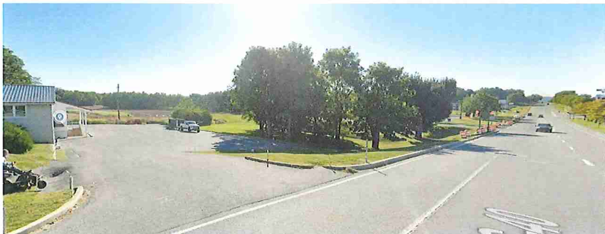
Photo 4: View along Dual Highway, looking southeast, showing the 100-year floodplain area.
