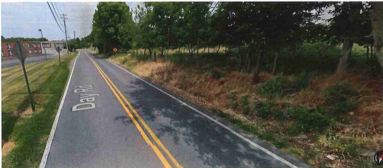
Photo 1: View north along Day Road, area to be rezoned to the right of the road.
