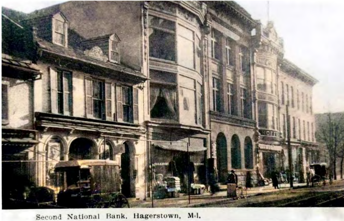
Historic postcard photo of the Myers and Eyerly buildings on West Washington Street, depicting multiple adjoining buildings displaying a variety of architectural elements. (Public Domain Photo)
