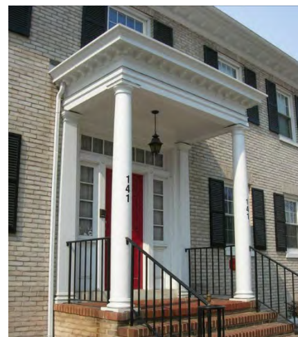
This replacement porch was constructed onto the front of a 19th Century home that was subject to major facade changes before the downtown historic district was created. Nonetheless, the owner created a new porch that is architecturally consistent with the nature of the home. (Staff Photo)
