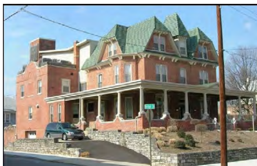
Corner property on North Potomac Street showing retaining walls along two streets. (Staff Photo)
