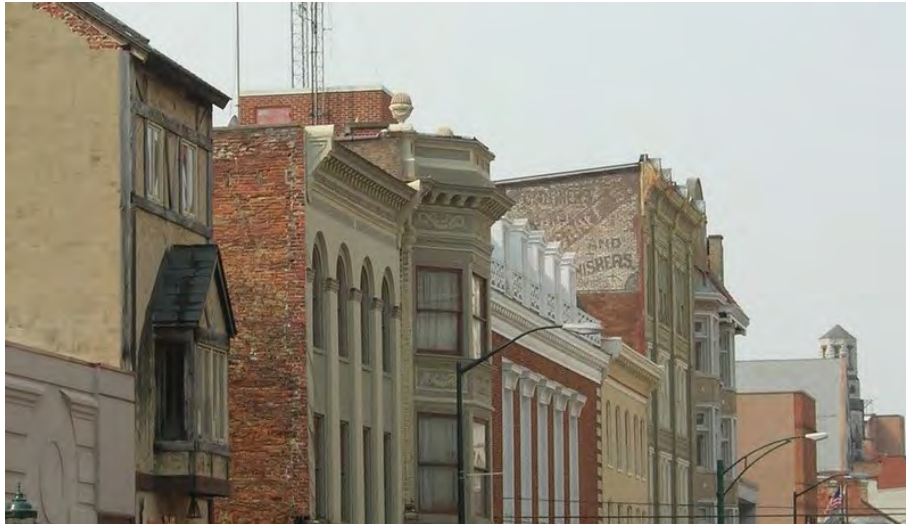
A variety of roof shapes define Hagerstown's skyline. (Staff Photo)
