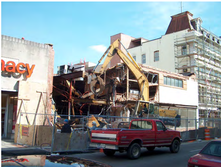
Demolition occurred in 2002 for the construction of University Plaza. The former Baldwin House Hotel is shown to the right, undergoing renovation to become the University System of Maryland Hagerstown Campus. Since its inception, the Historic District Commission has approved over 90% of the demolition applications submitted for review. (Staff photo)
