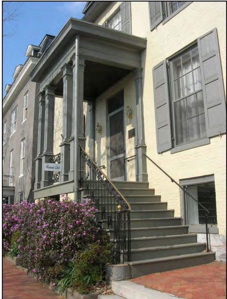
The Women's Club on South Prospect Street (Staff Photo)
