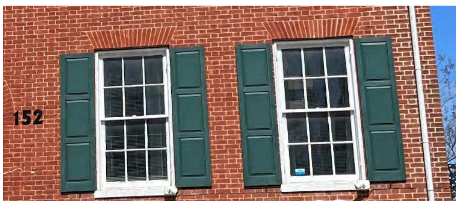
First floor shutters on the Congressman Roman House (also known as the Kneisley Building) on West Washington Street. Congressman James Roman led the local effort to meet Confederate demands during the "Ransom of 1864". (Staff Photo)
