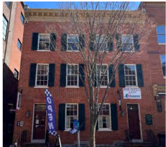
Differences in masonry patterns on the front of this building reveal that the third floor was added at some time after the building's original construction. (Staff Photo)
