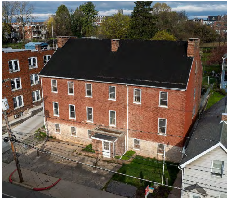
The Washington County Almshouse ( Staff photo )
