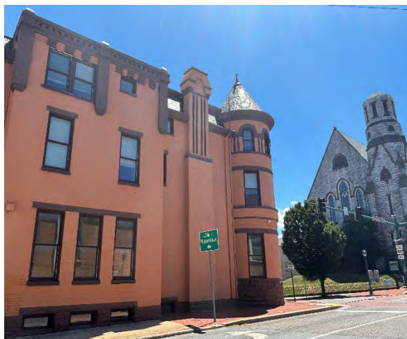
Ornate chimney on the Richardsonian Romanesque house on West Washington Street (Staff photo)
