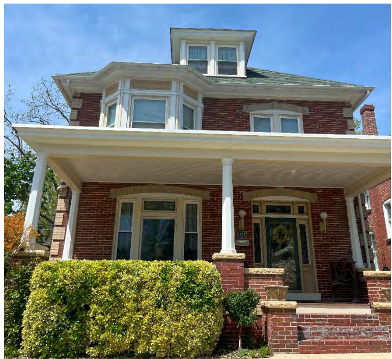
American Foursquare-style house at 903 Potomac Avenue (Staff Photo)
