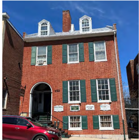
The Federal/Neoclassical-style Kneisley Building at 152 West Washington Street (Staff photo)
