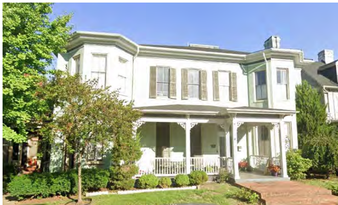
When available, use historic evidence when reconstructing porches on contributing structures. (Staff photo)
