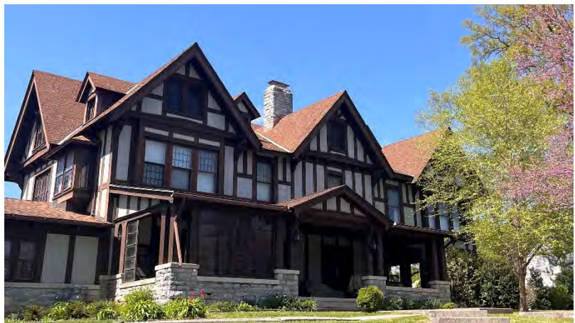
Tudor Revival-style house at 815 The Terrace ( Staff Photo )
