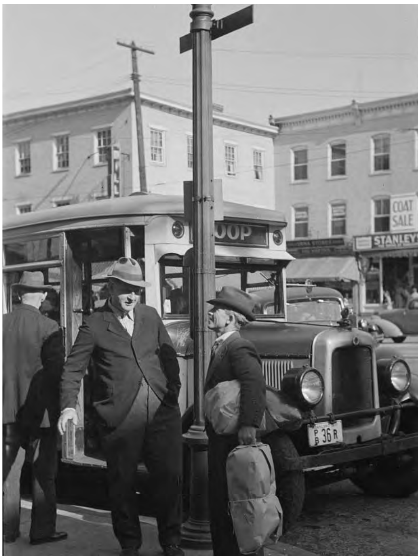
A summer Sunday afternoon shopping in downtown Hagerstown, circa 1938. The early 19 th Century mixed use buildings in the background, and others to the left of this photo have iconically framed the north side of Public Square for approaching two centuries. (Library of Congress photo)
