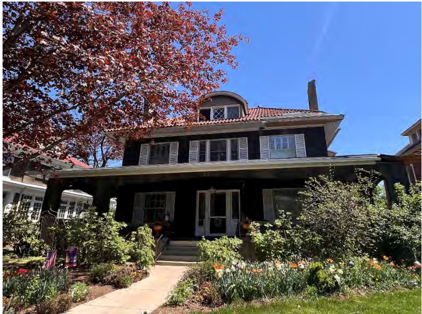
Mission Revival-style house at 810 Oak Hill Avenue (Staff Photo)
