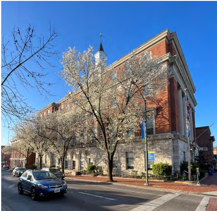
City Hall with East Franklin Street to the left (Staff Photo)
