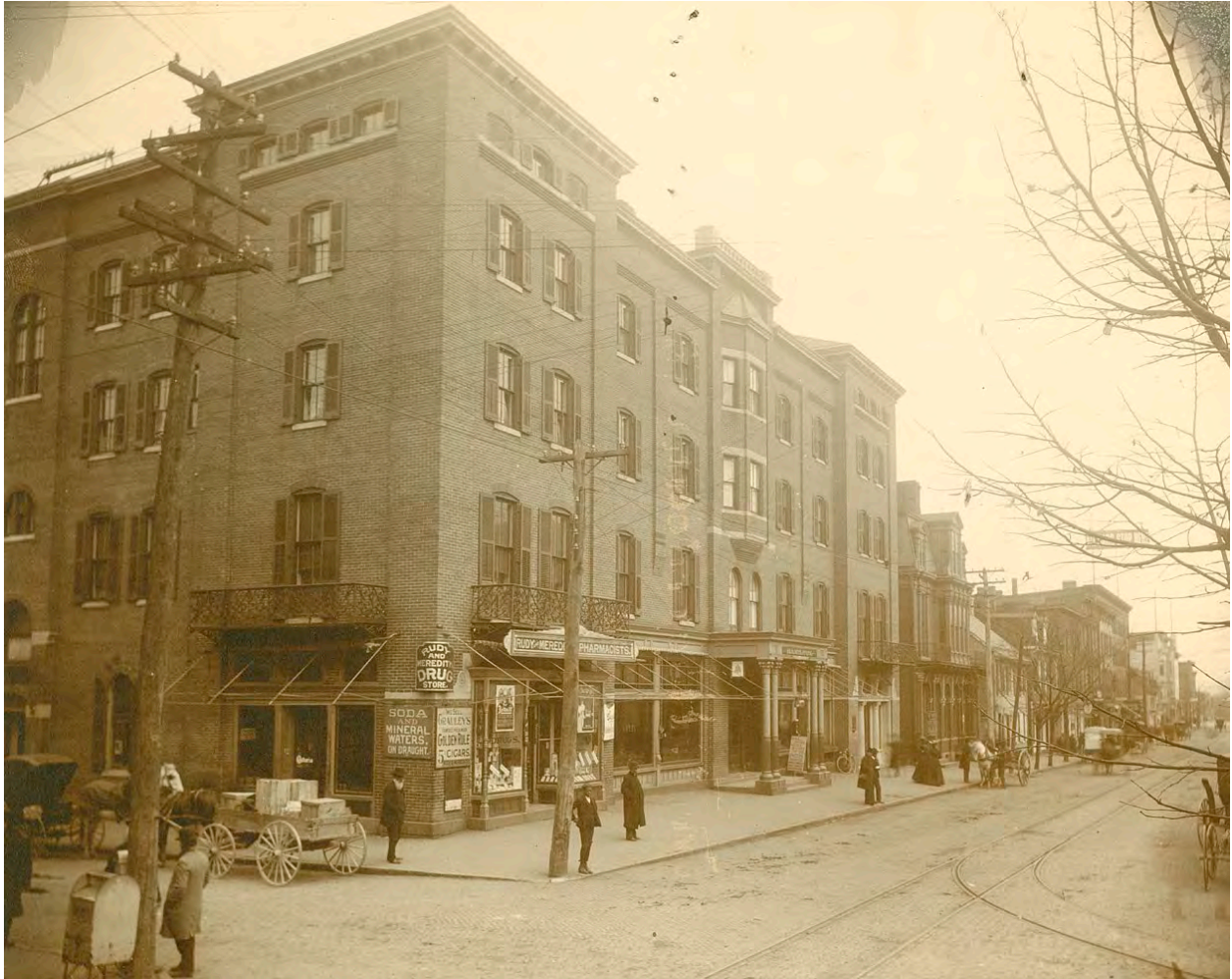
The Hamilton Hotel, circa 1905. The Hamilton was constructed in 1888 by former Maryland Governor and U.S. Senator William T. Hamilton, who was a Hagerstown resident. The building was recently renovated for commercial and residential apartment use (Washington County Historical Society Photo)
