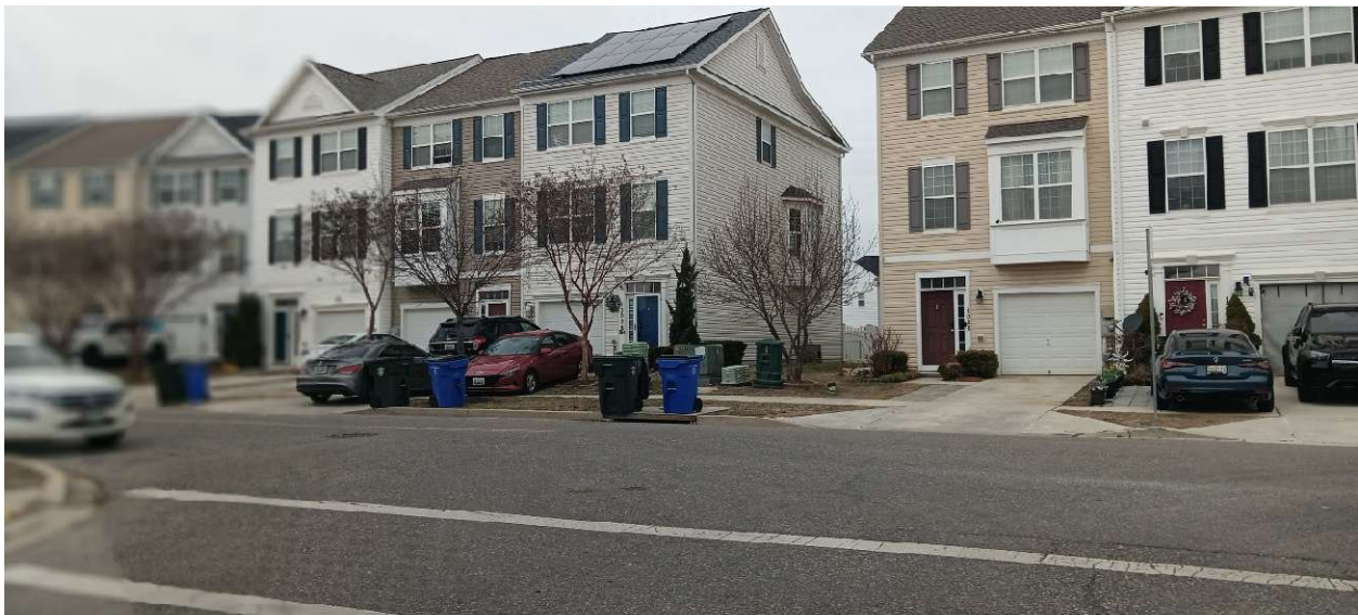
Yellow Jacket Road, Collegiate Acres, Hagerstown. Townhouse on right shows owner paved entire front yard with pavers, drives over grassed area at driveway apron, and barely misses a street sign in the very small area between the two driveway aprons.
