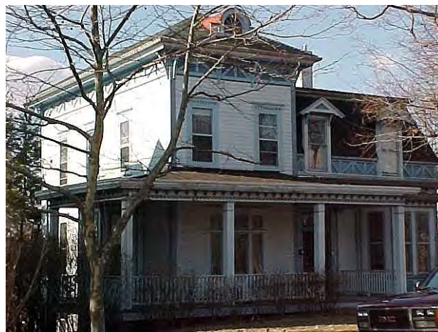
Eastern Stick-style house at 121 S Prospect Street (Staff Photo)
