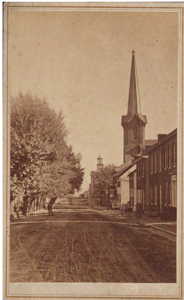
West Franklin Street, viewed to the east from approximately in front of today's United States Post Office building, circa 1875. Trinity Lutheran Church is seen at right. The church later relocated to North Potomac Street. Town Hall is seen in the background with the clock and bell tower. Although not seen here due to distance and lighting, the city's iconic "Little Heiskell" weather vane stood atop the town hall bell tower. Notice how street trees stood only on the left (north) side of the street, protecting the south-facing fronts of those buildings from the heat of the sun. The front (north) side of the buildings on the right did not receive direct sunlight. This photo was captured by pioneering local photographer Elias Recher. ( Library of Congress Photo )
