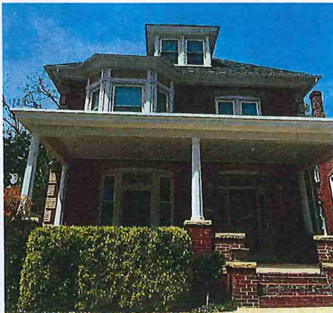
American Foursquare-style house at 903 Potomac Avenue (Staff Photo)
