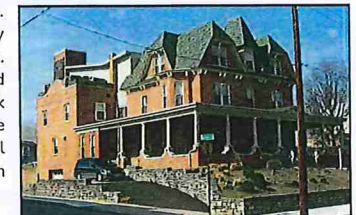
Corner property on North Potomac Street showing retaining walls along two streets. (Staff Photo)
