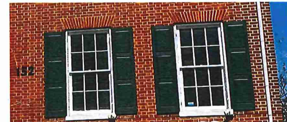
First floor shutters on the Congressman Roman House (also known as the Kneisley Building) on West Washington Street. Congressman James Roman led the local effort to meet Confederate demands during the "Ransom of 1864". (Staff Photo)
