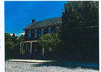
Middlekauff House (Staff photo)
