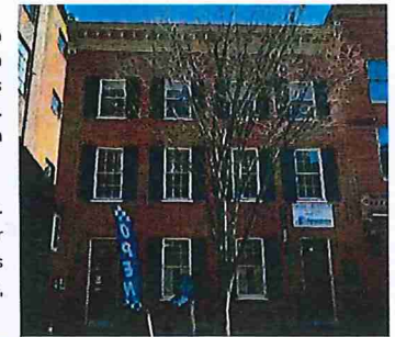
Differences in masonry patterns on the front of this building reveal that the third floor was added at some time after the building's original construction. (Staff Photo)
