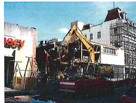
Demolition occurred in 2002 for the construction of University Plaza. The former Baldwin House Hotel is shown to the right, undergoing renovation to become the University System of Maryland Hagerstown Campus. Since its inception, the Historic District Commission has approved over 90% of the demolition applications submitted for review. (Staff photo)
