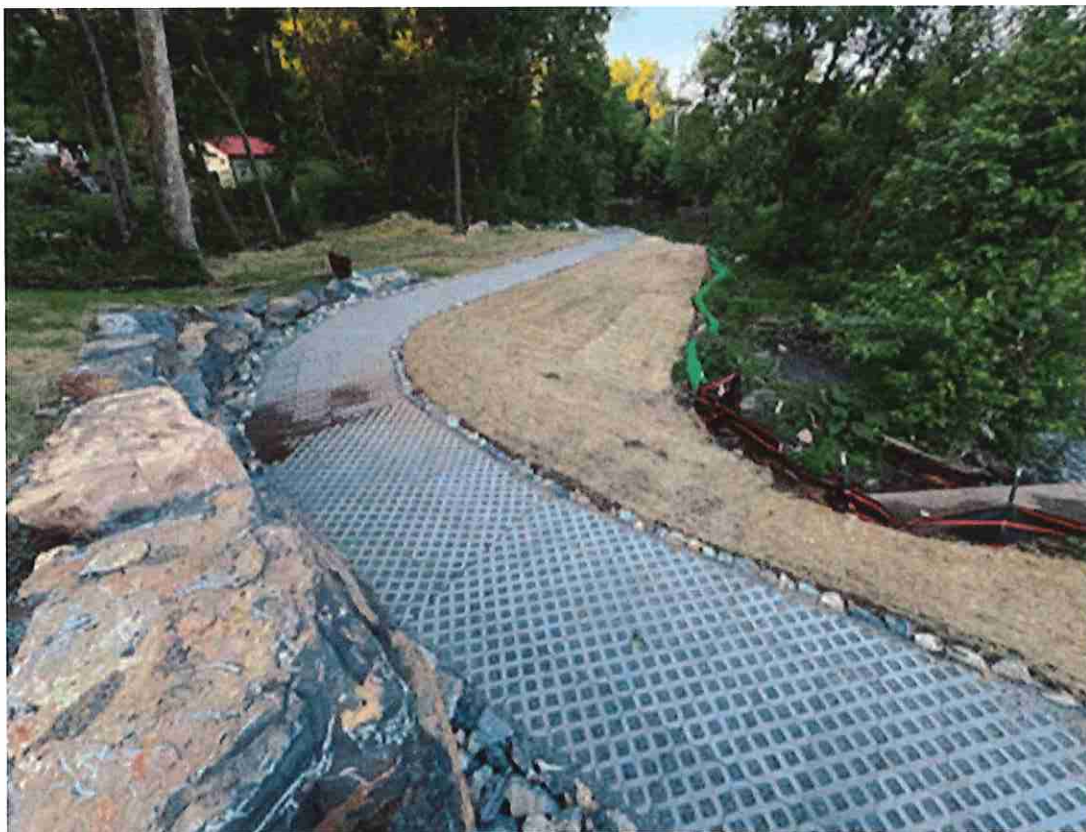
Looking down the downstream side of the trail leading to the water. The end of the dam is visible to the right of the photo.
