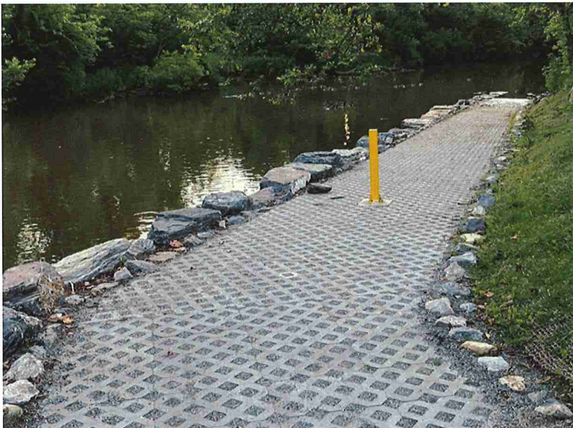
Looking upstream at Antietam Creek. Access to the water is easily available down a long, gentle slope to the water. A yellow bollard prevents vehicles from attempting to use the ramp. Access is for those using small watercraft such as kayaks and canoes.
