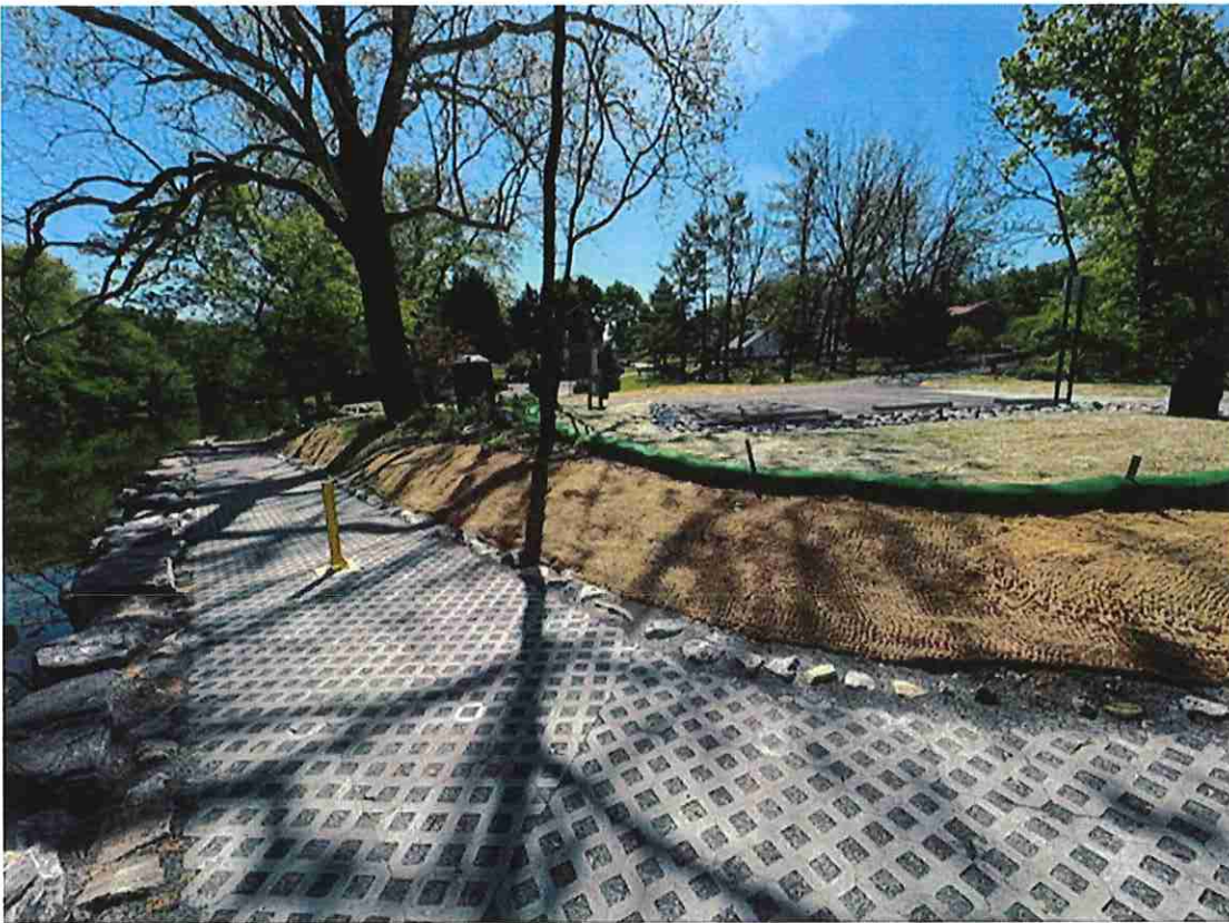
Looking east towards the parking lot with the upstream ramp to the left of the photo.
