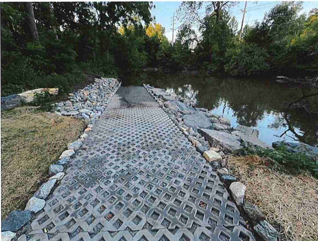
Looking at the downstream access ramp.
