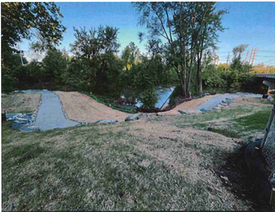
A view of the downstream portion of the trail as it winds around the dam.
