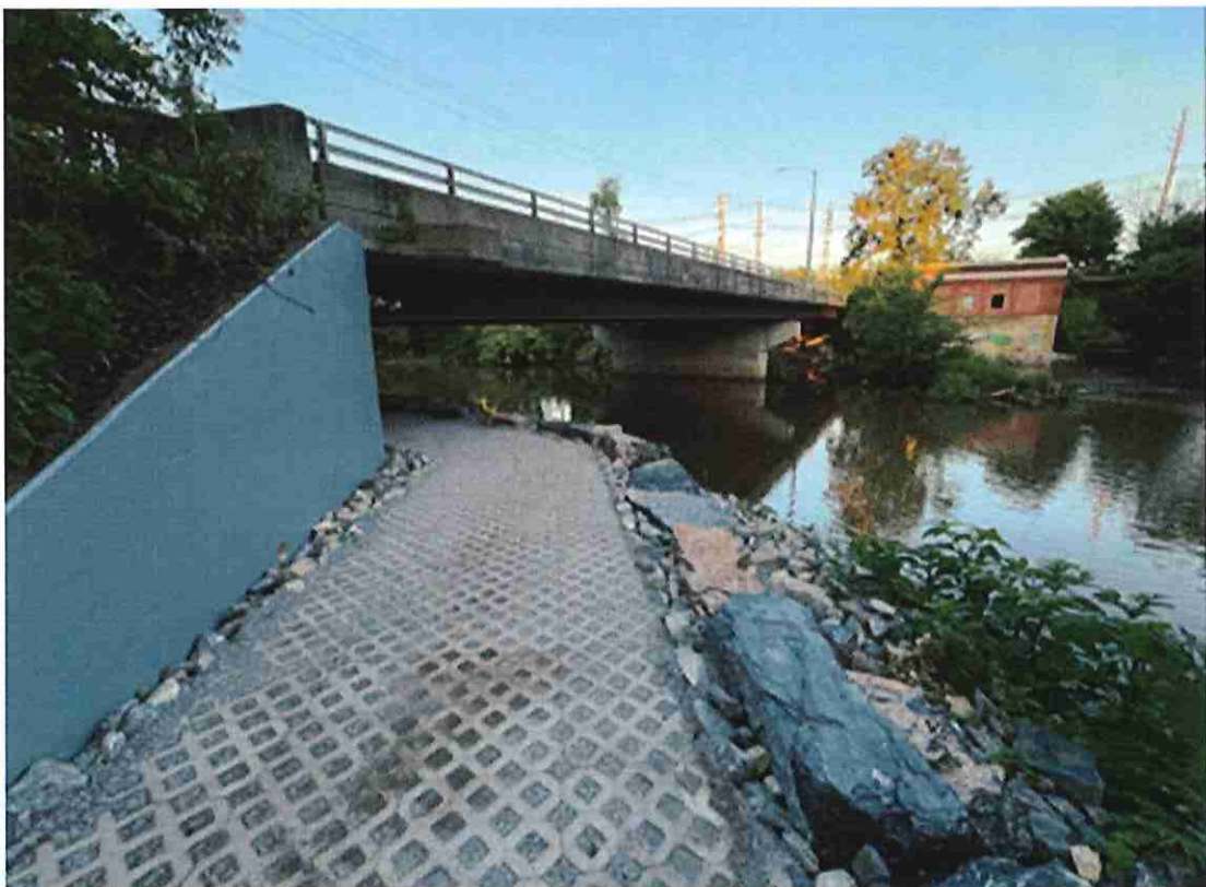
The downstream trail takes visitors under the Mt. Aetna Road bridge. Remnants of the former electrical power plant can be seen to the right.
