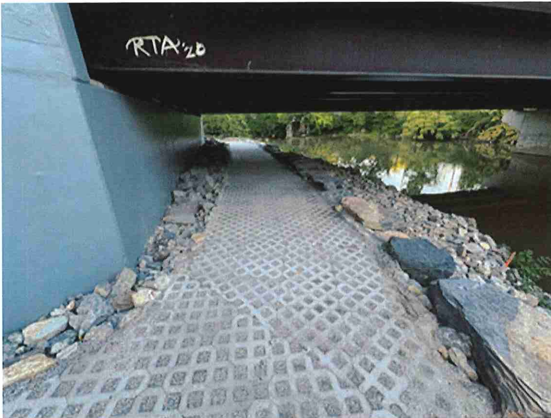
Looking downstream as the trail extends beneath the bridge itself.
