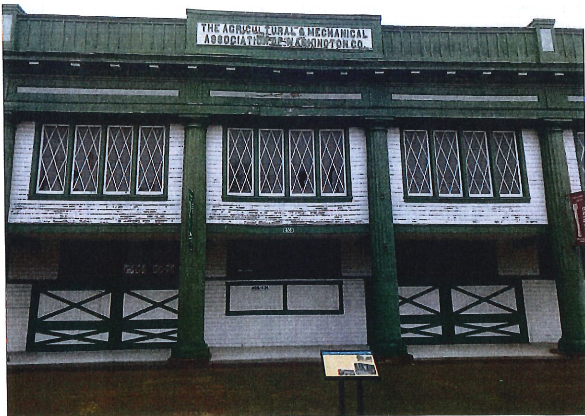
Front Face of Entrance Building
