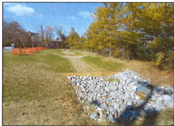
Figure 6 – Stormwater Retrofit Projects Bioswale installed at Hager Park.
