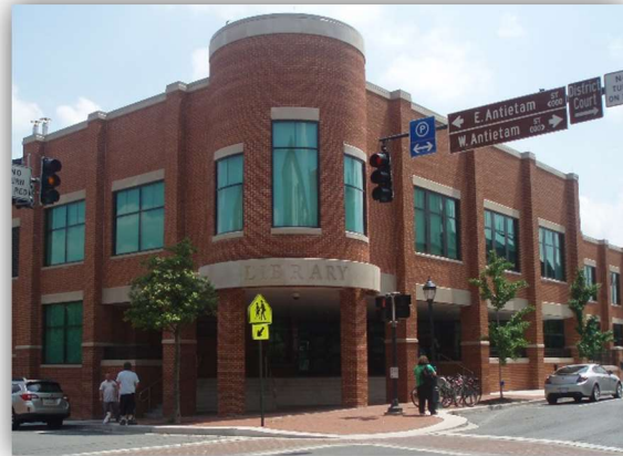
Central Library at S. Potomac St & W. Antietam St
