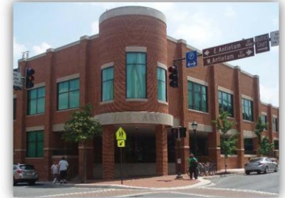
Central Library at S. Potomac St & W. Antietam St
